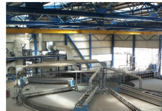
UCEGO NO. 12 A Under assembly – general view
