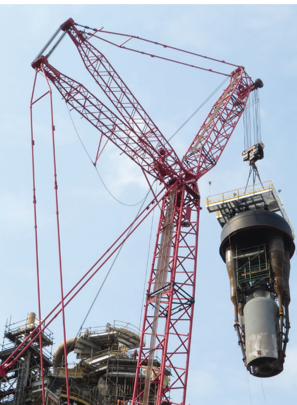
Installation of this riser termination device in the reactor reduced coke and dry gas and improved product yield selectivity.
