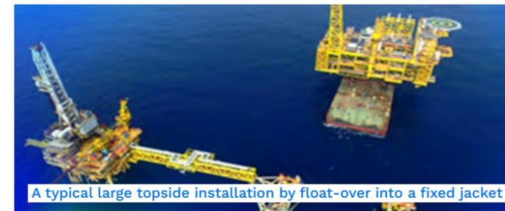
A typical large topside installation by float-over into a fixed jacket
