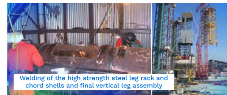
Welding of the high strength steel leg rack and chord shells and final vertical leg assembly
