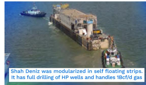
Shah Deniz was modularized in self floating strips. It has full drilling of HP wells and handles 1Bcf/d gas
