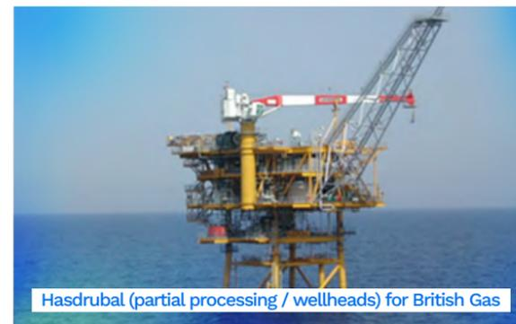
Hasdrubal (partial processing / wellheads) for British Gas
