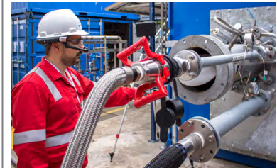
T.EN burner test facility
