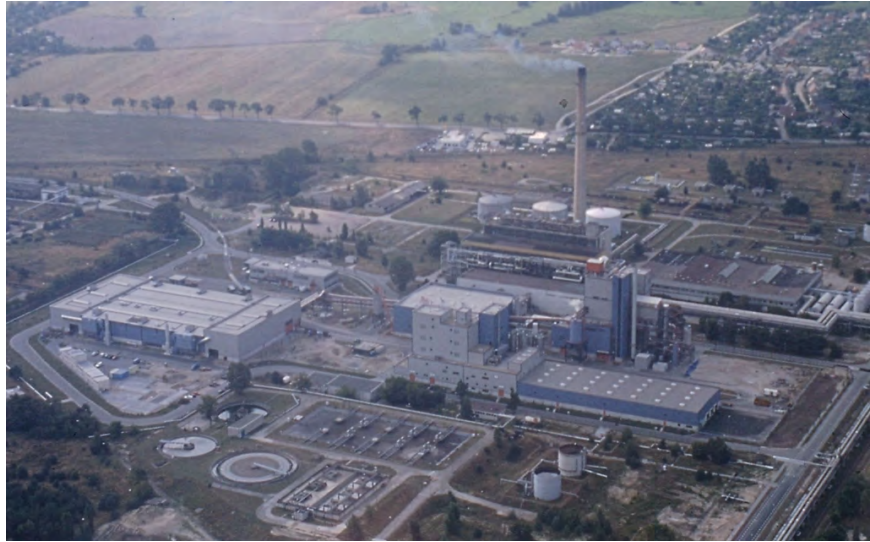
PA 6 plant with solid waste recycling
