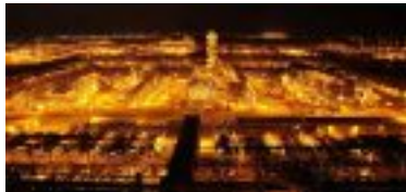
Khursaniyah Gas Plant, Kingdom of Saudi Arabia - 1 BSCFD CRYOMAX unit
