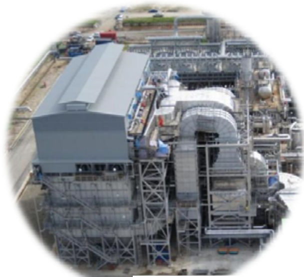
Large scale reformer
